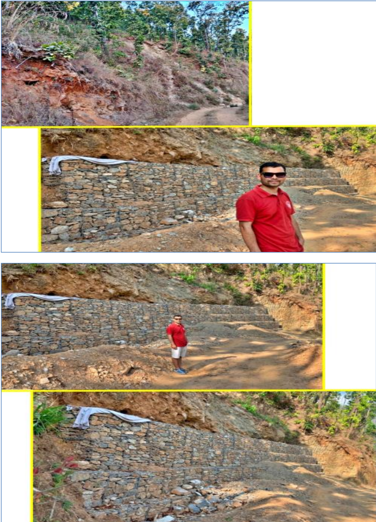
Figure 54: Tusara Chhipchipe Landslide Treatment
