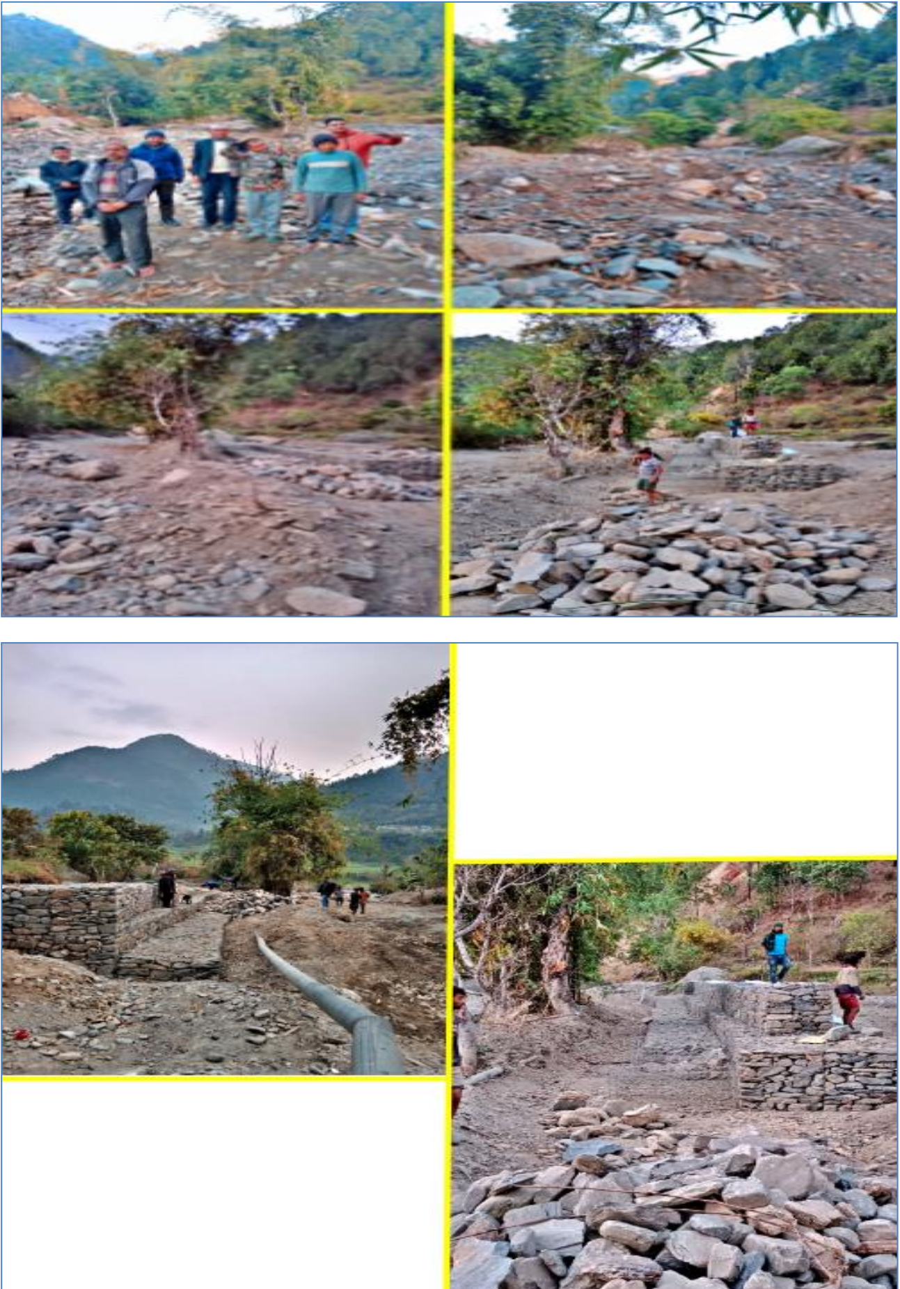
Figure 67: Chhatipata Lankuri Khola Stream Bank Protection
