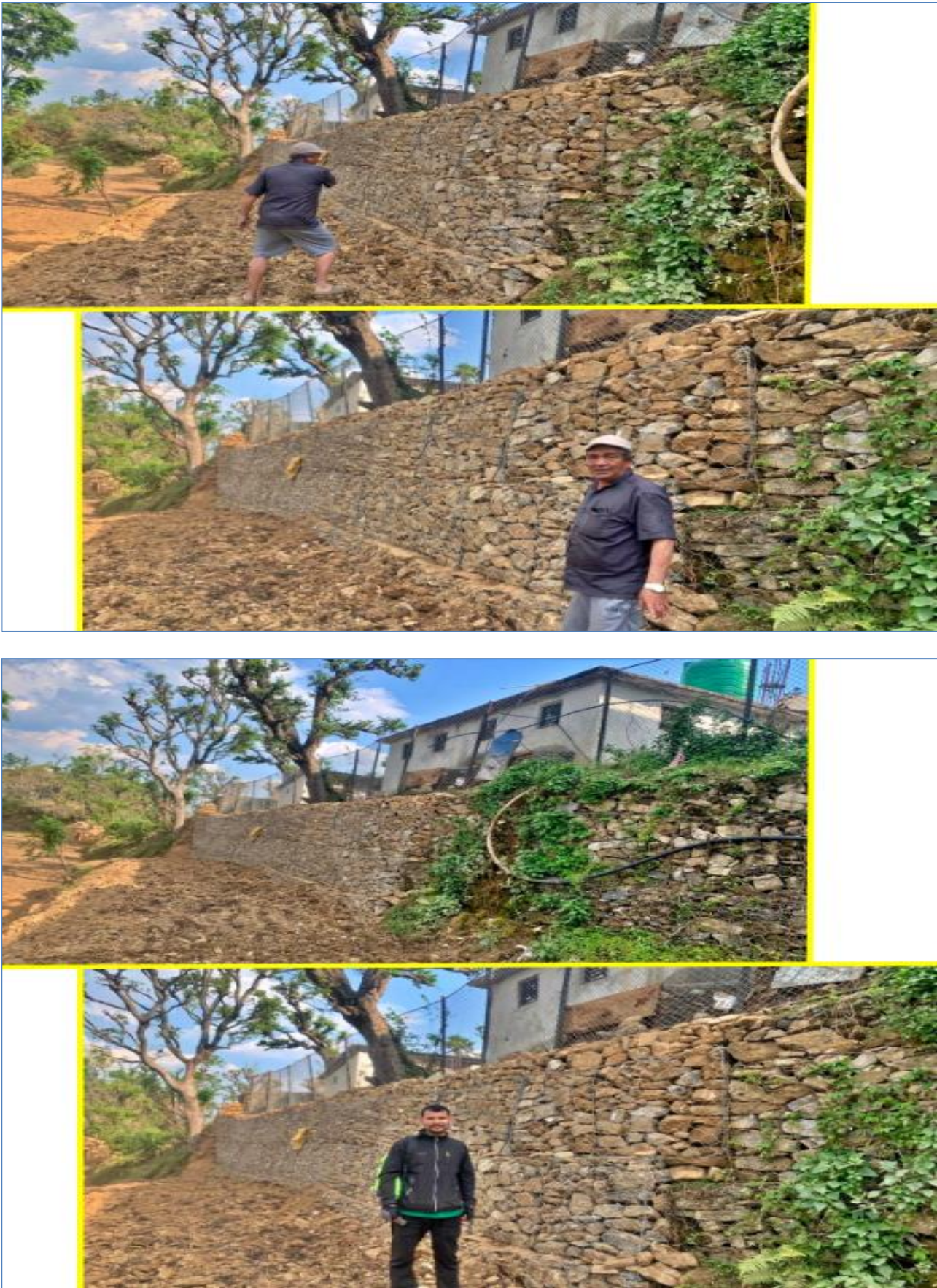
Figure 21: Gajul Landslide Treatment
