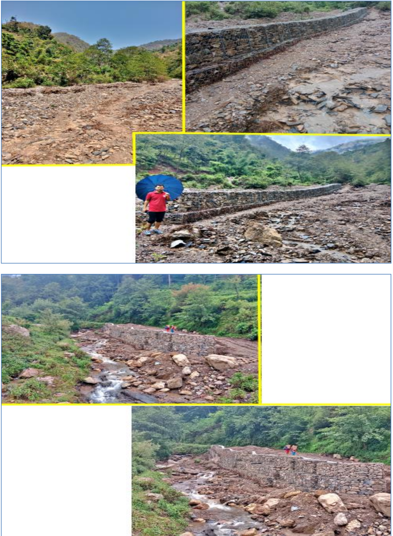
Figure 11: Laharikhola Torrent Control
