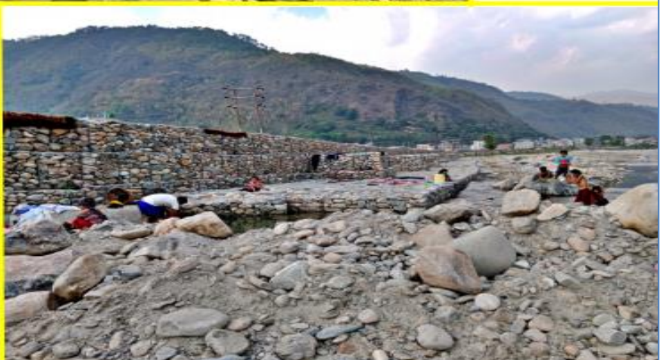
Figure 65: Jhimrukh River Bank Protection
