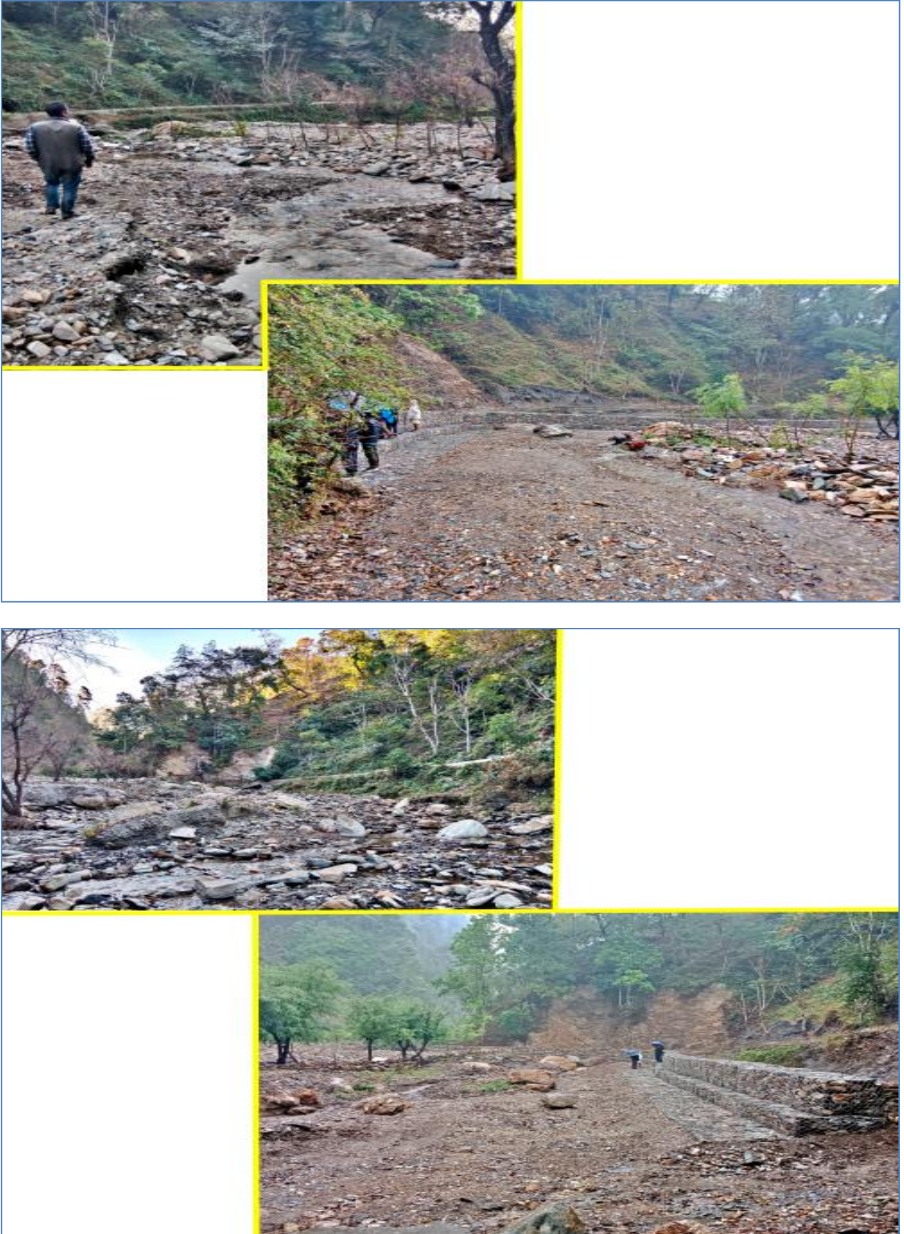
Figure 24: Jutung Khola Stream Bank Protection
