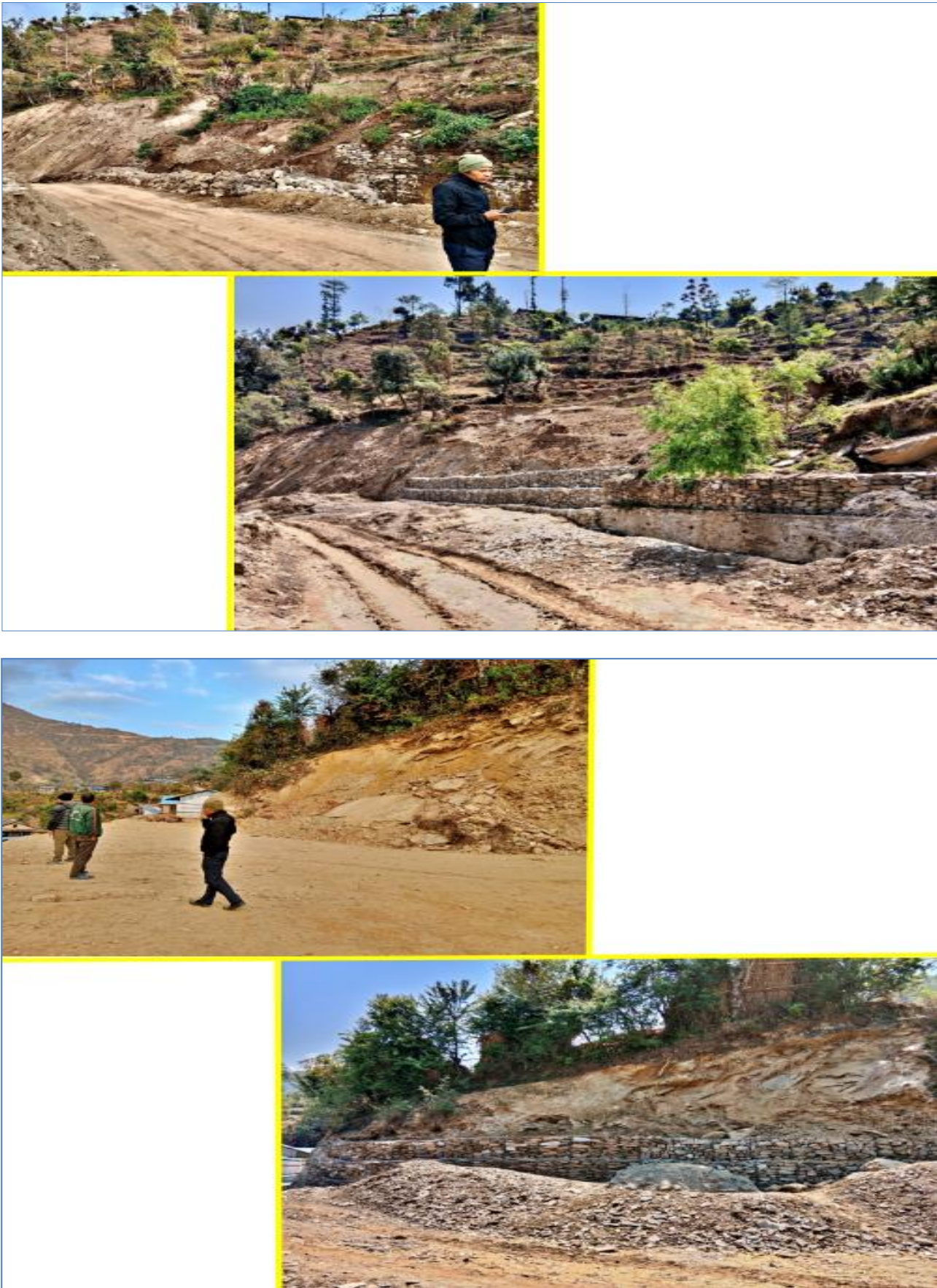
Figure 17: Sandada Landslide Treatment
