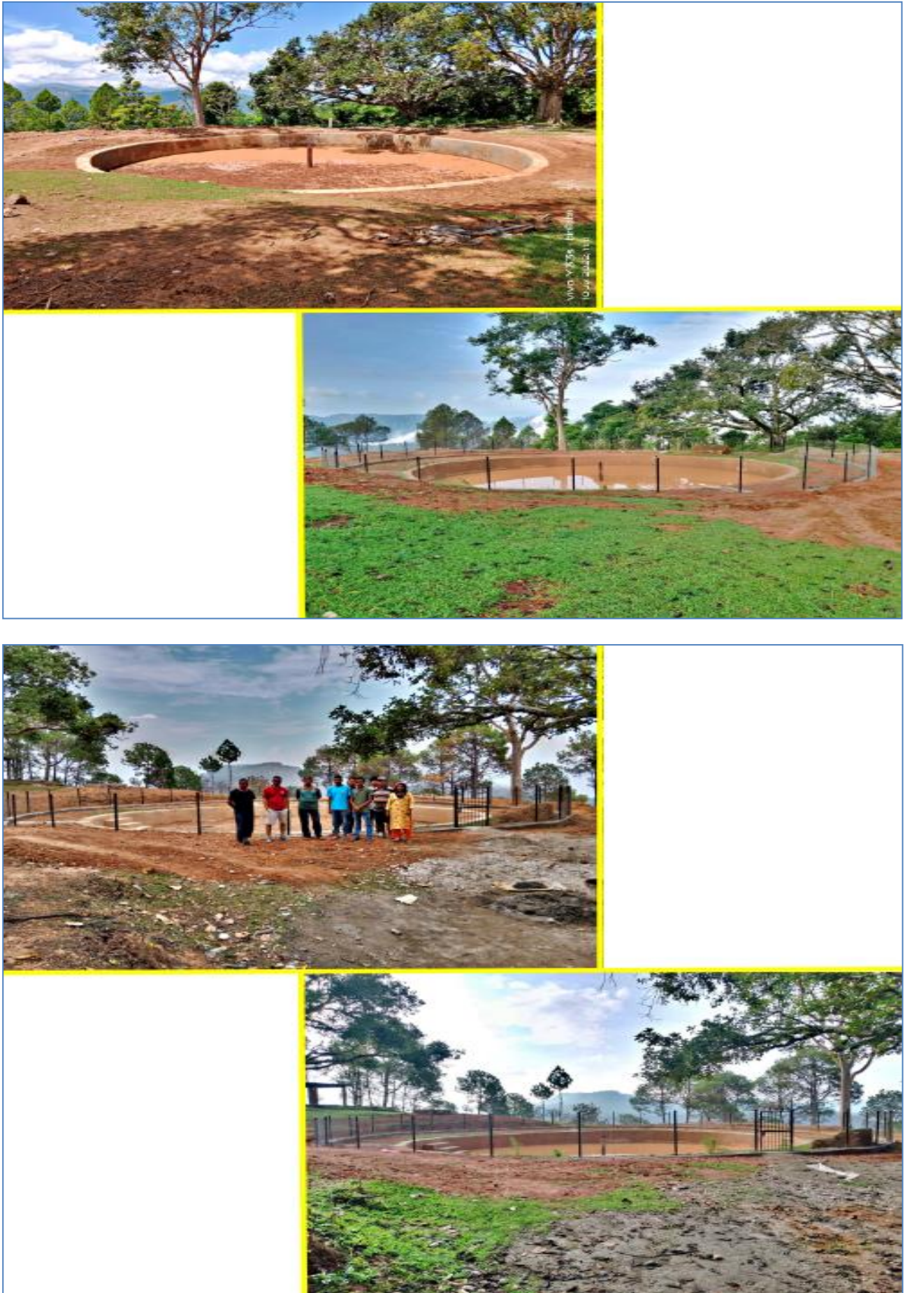
Figure 68: Khairakot Pond Maintenance & Fencing
