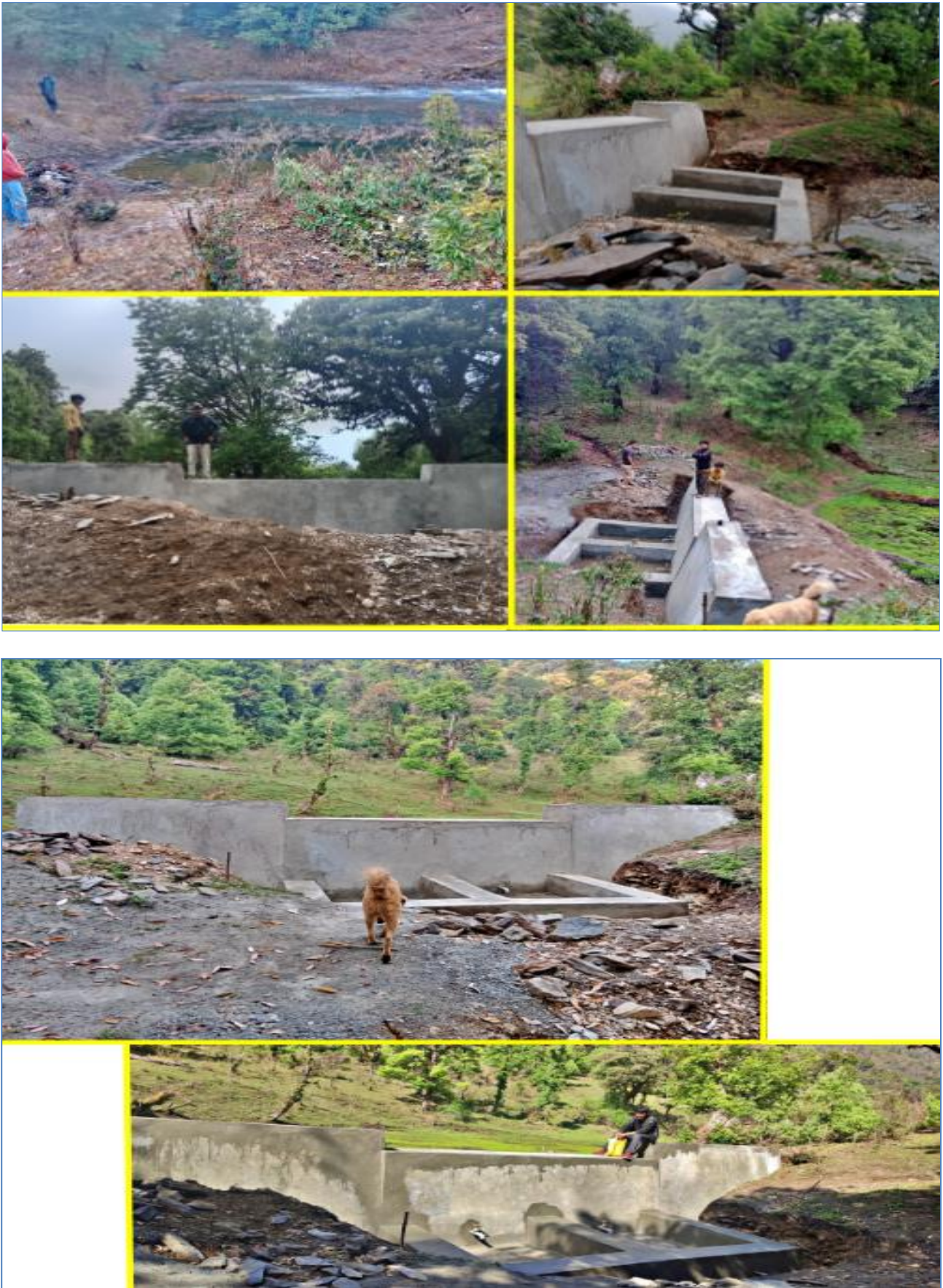
Figure 48: Ratodaha Protection Work
