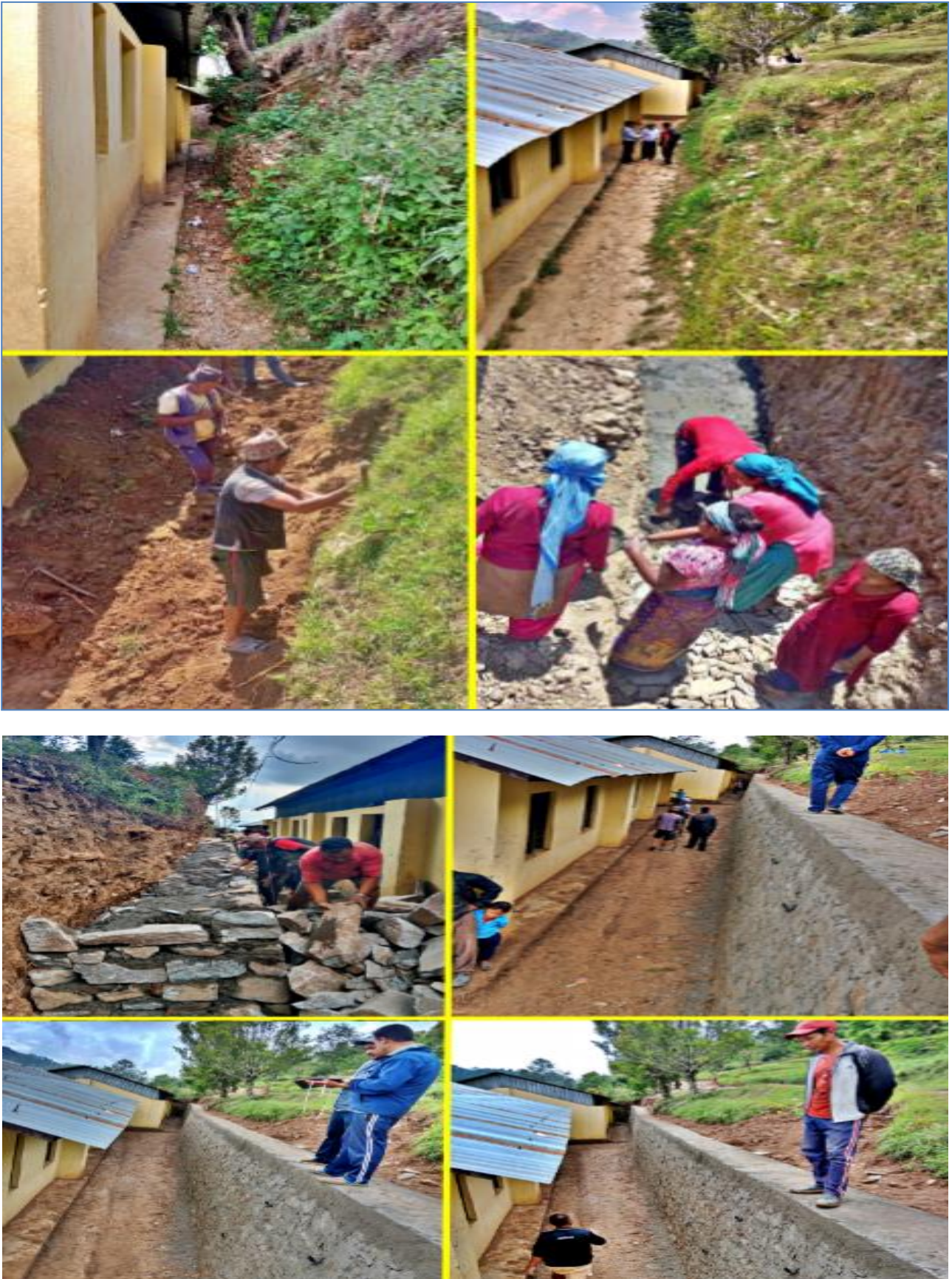
Figure 8: Bhanbhane Landslide Treatment
