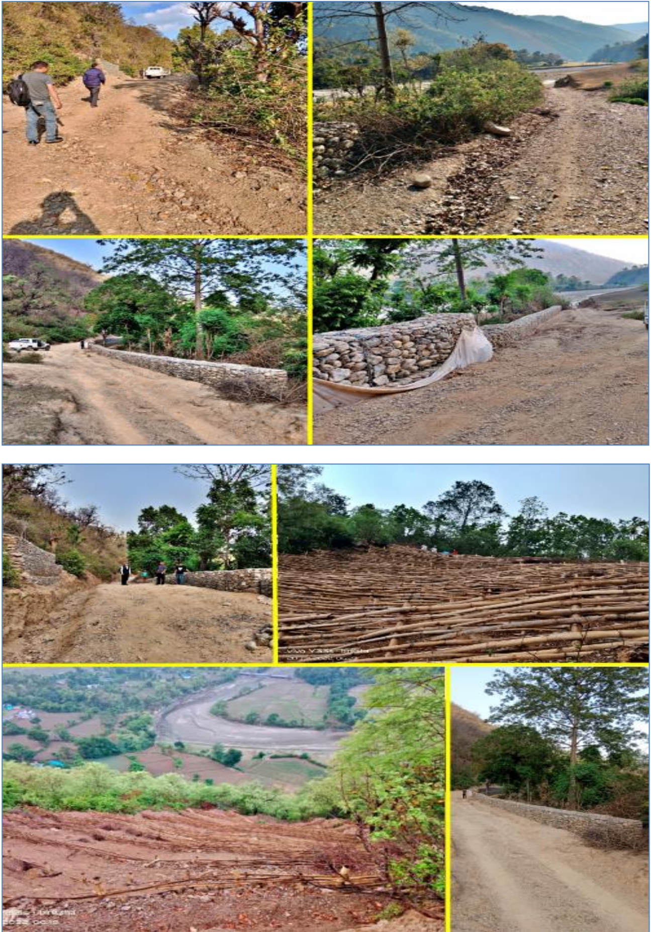
Figure 58: Siundada Landslide Treatment
