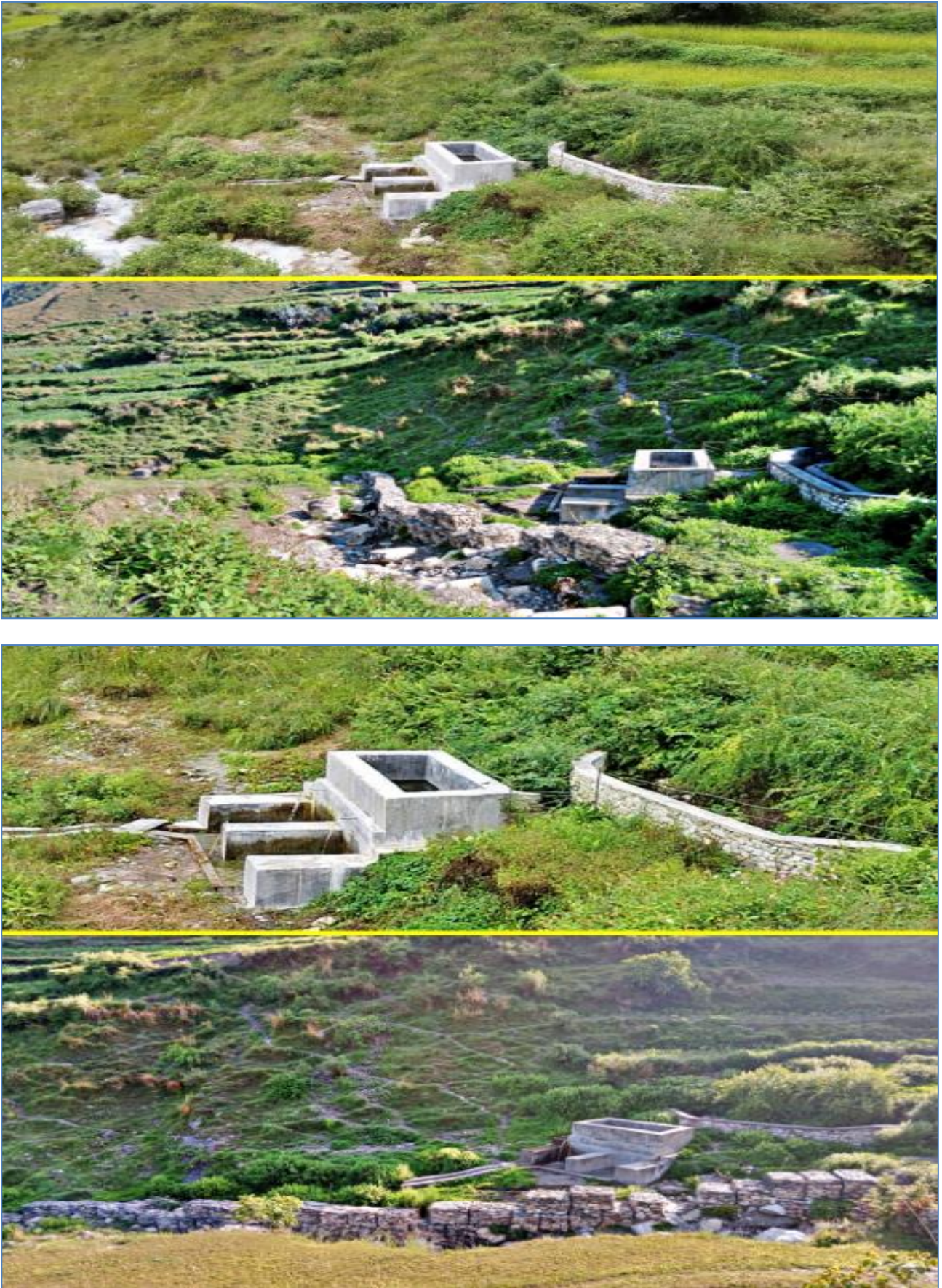
Figure 42: Maikot Torrent Control
