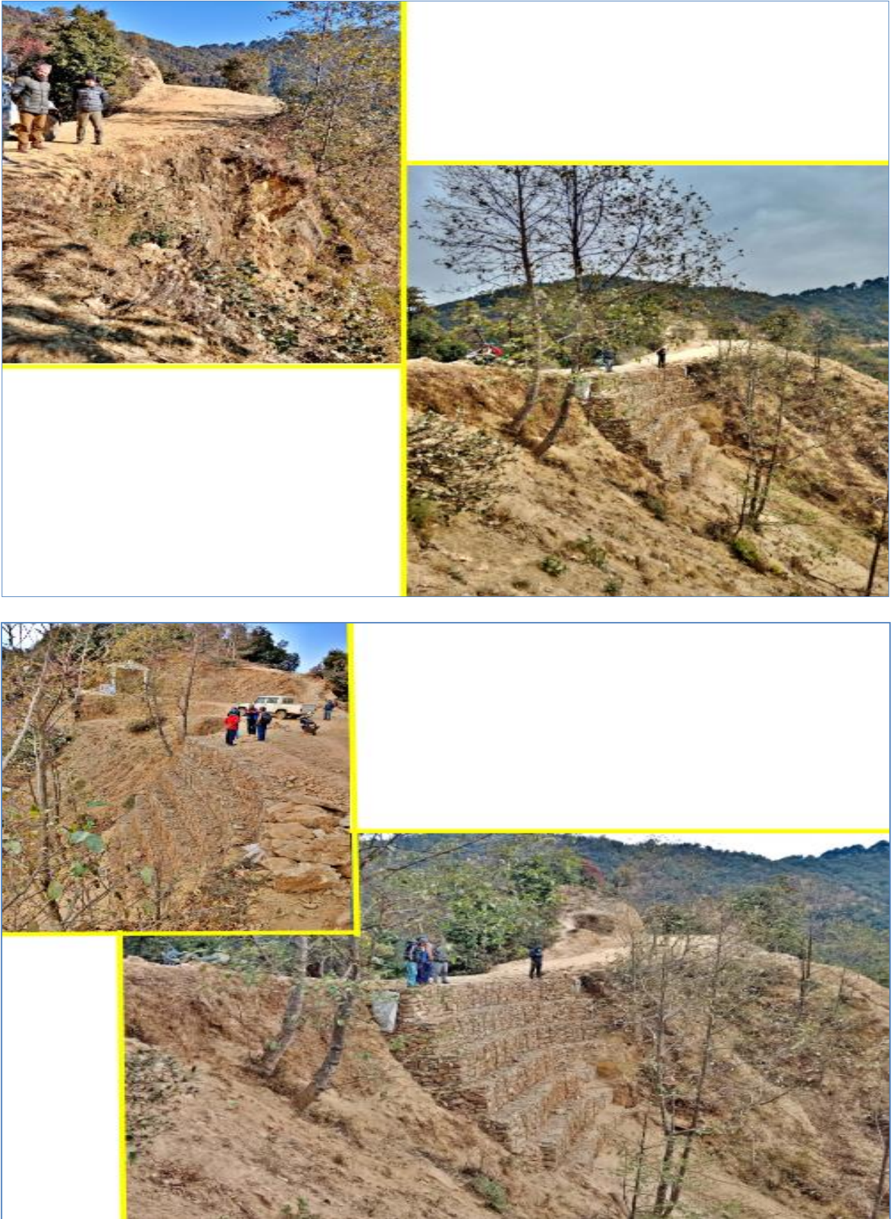
Figure 18: Tarikhola Landslide Treatment
