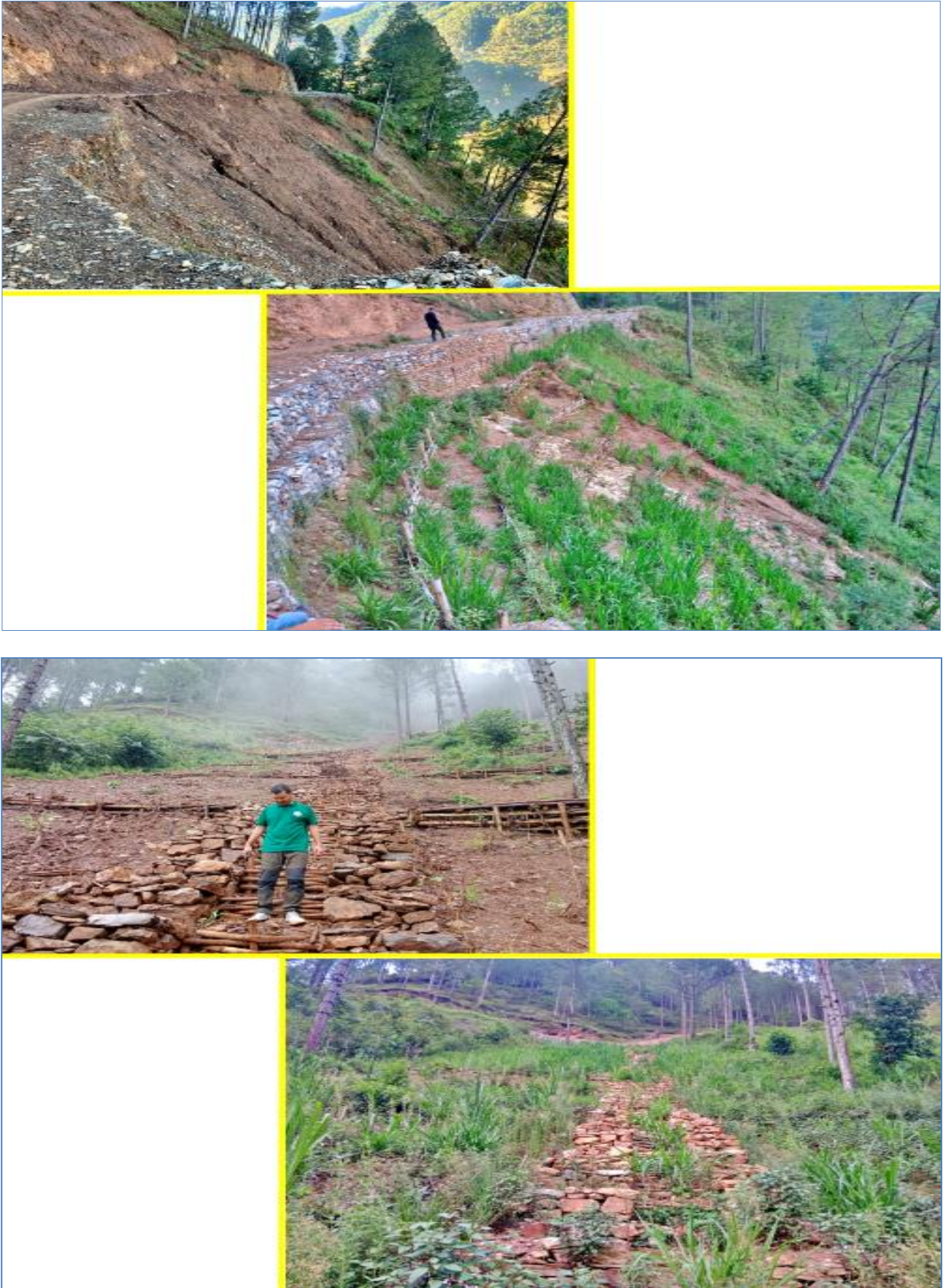
Figure 39: Bamboo Crib Wall, Fascine, Wattling Construction
