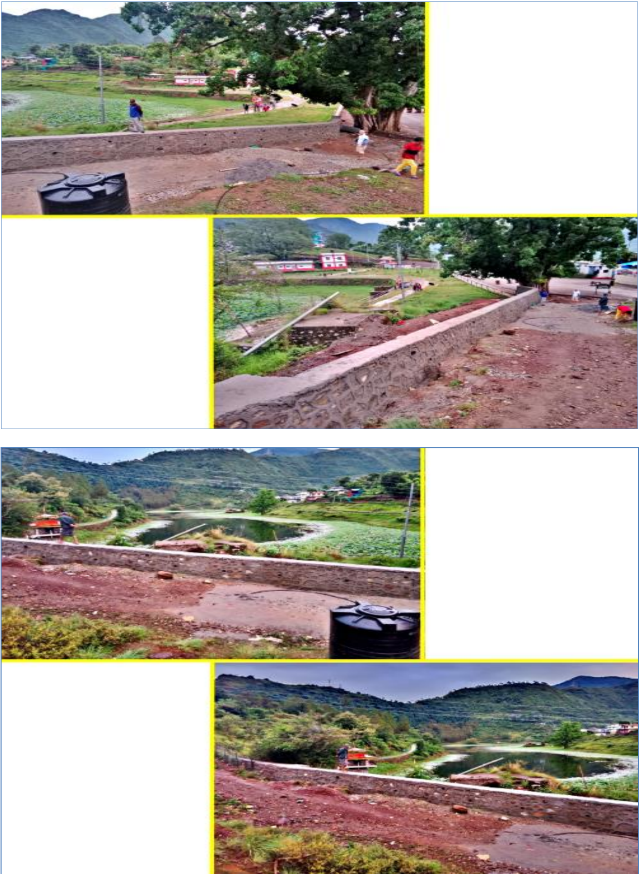
Figure 47: Kamaldaha Protection Work
