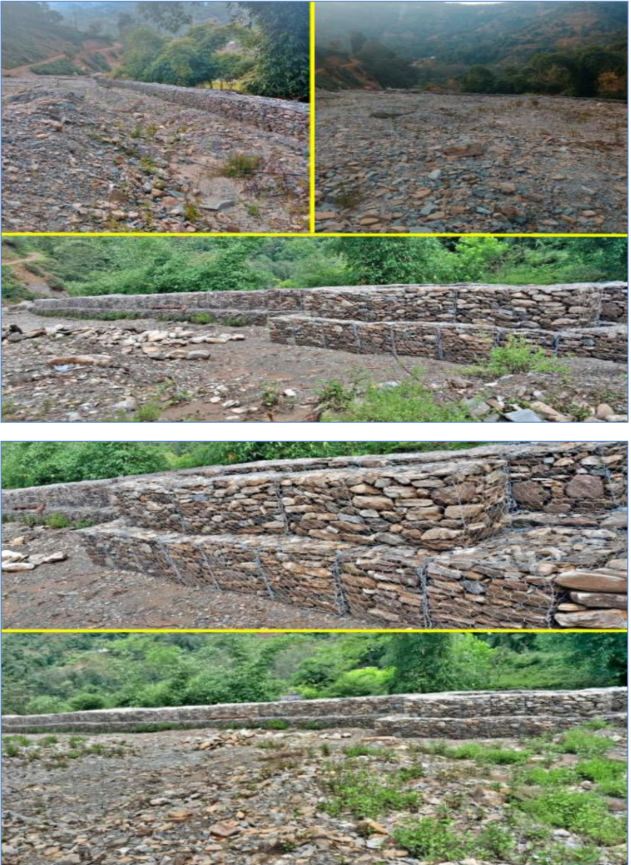
Figure 9: Bhoksiwang Dhangsi Khola Torrent Control
