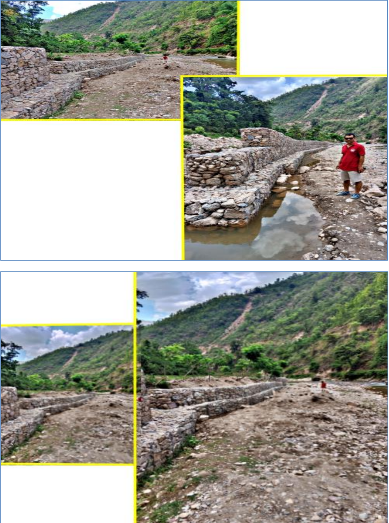
Figure 22: Sulibagar Madikhola Landslide Treatment
