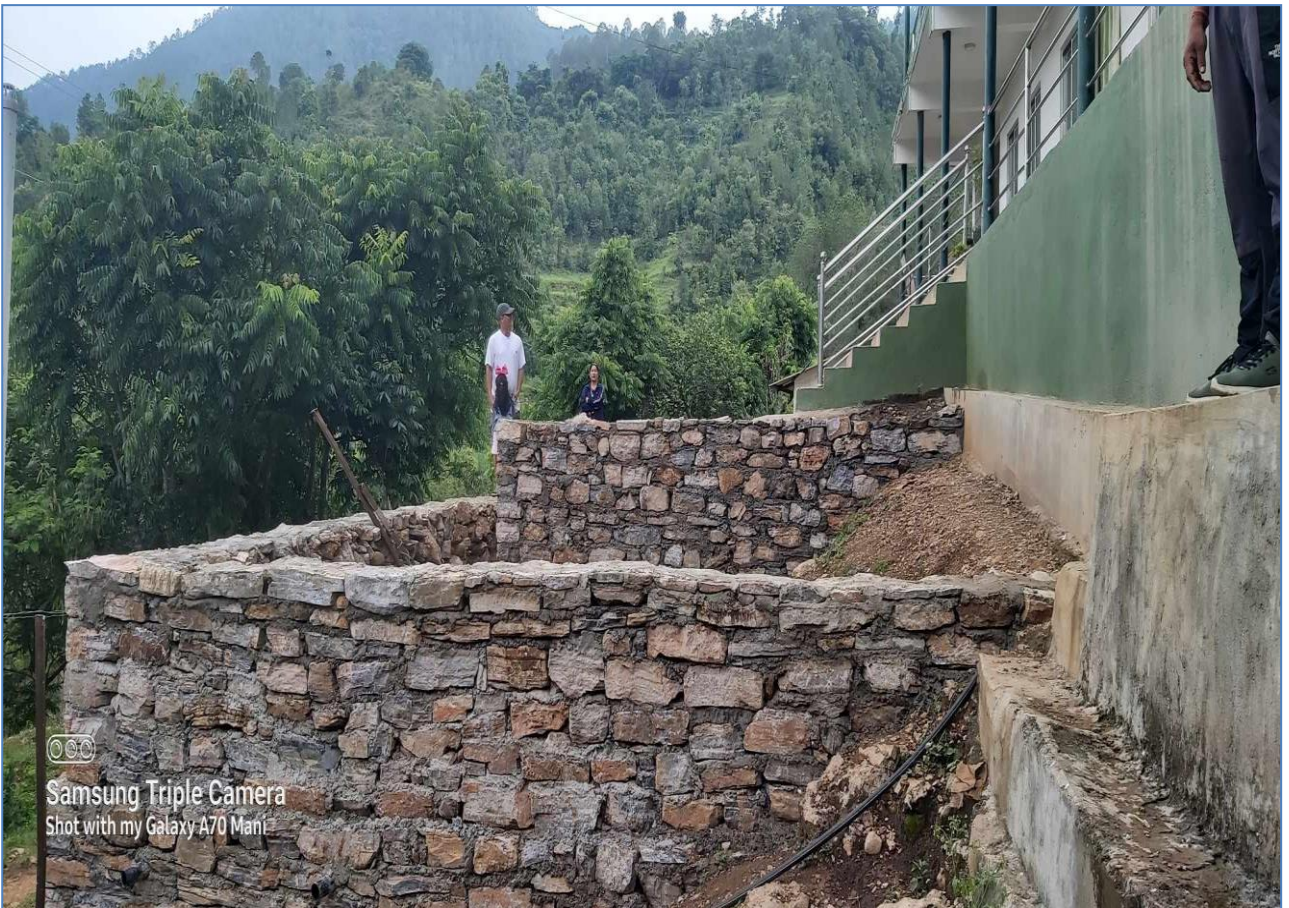
Figure 35: Barreck Landslide Treatment
