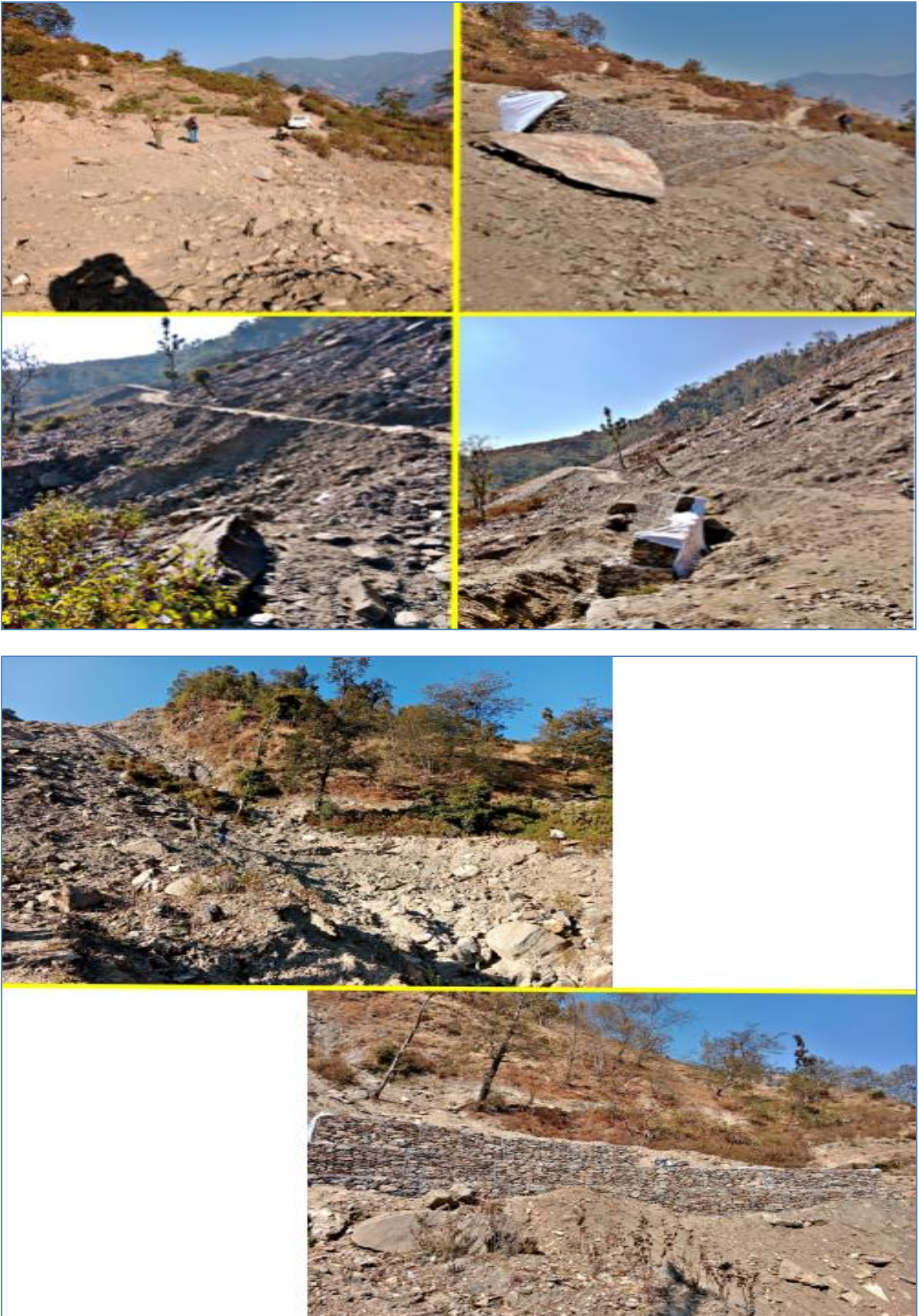
Figure 61: Jugekhola Landslide Treatment
