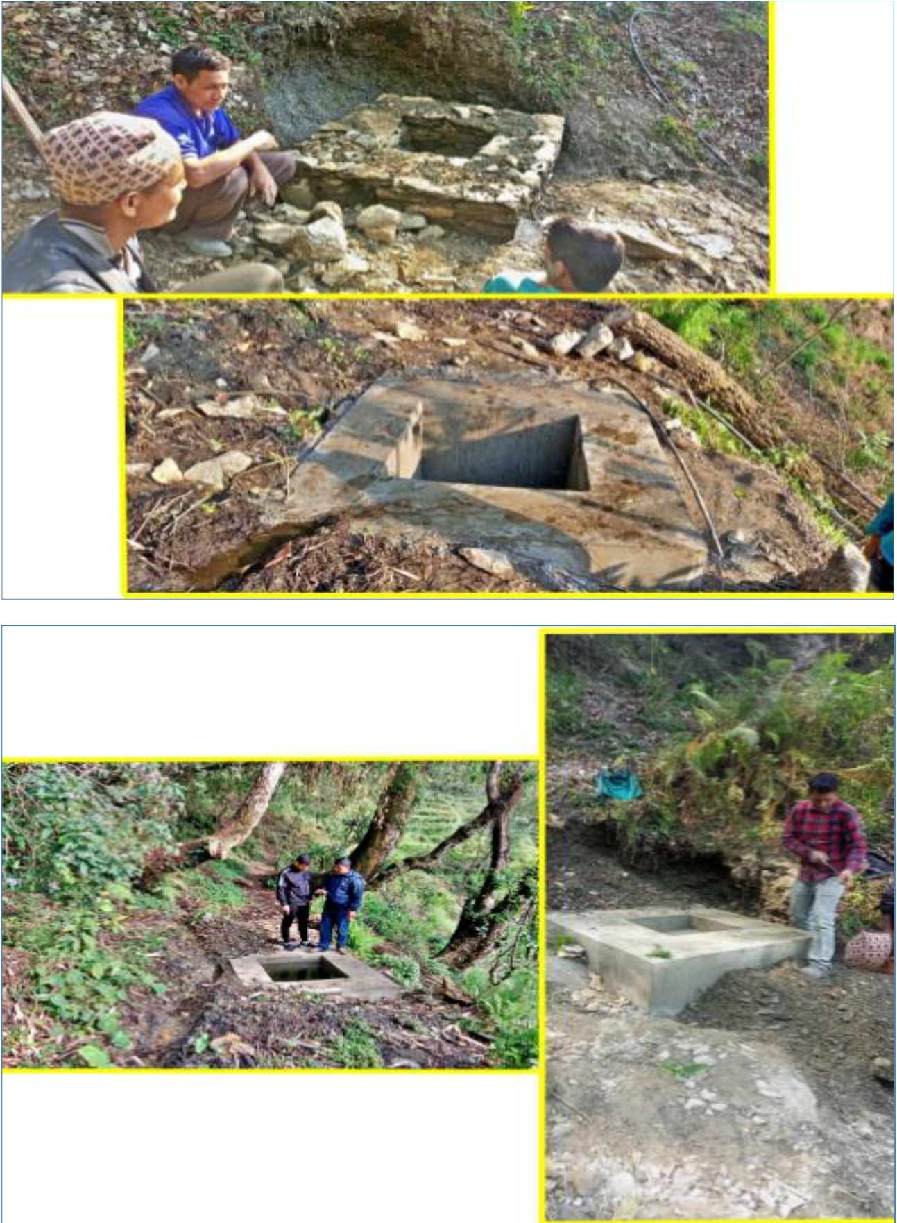
Figure 37: Bhanbhane Water Source Protection
