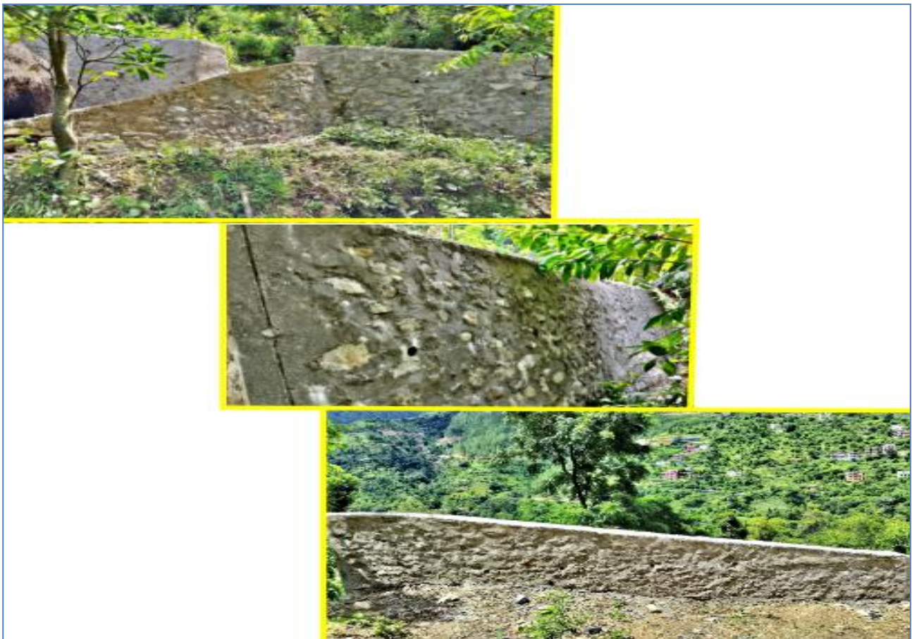
Figure 12: Runtawang Landslide Treatment
