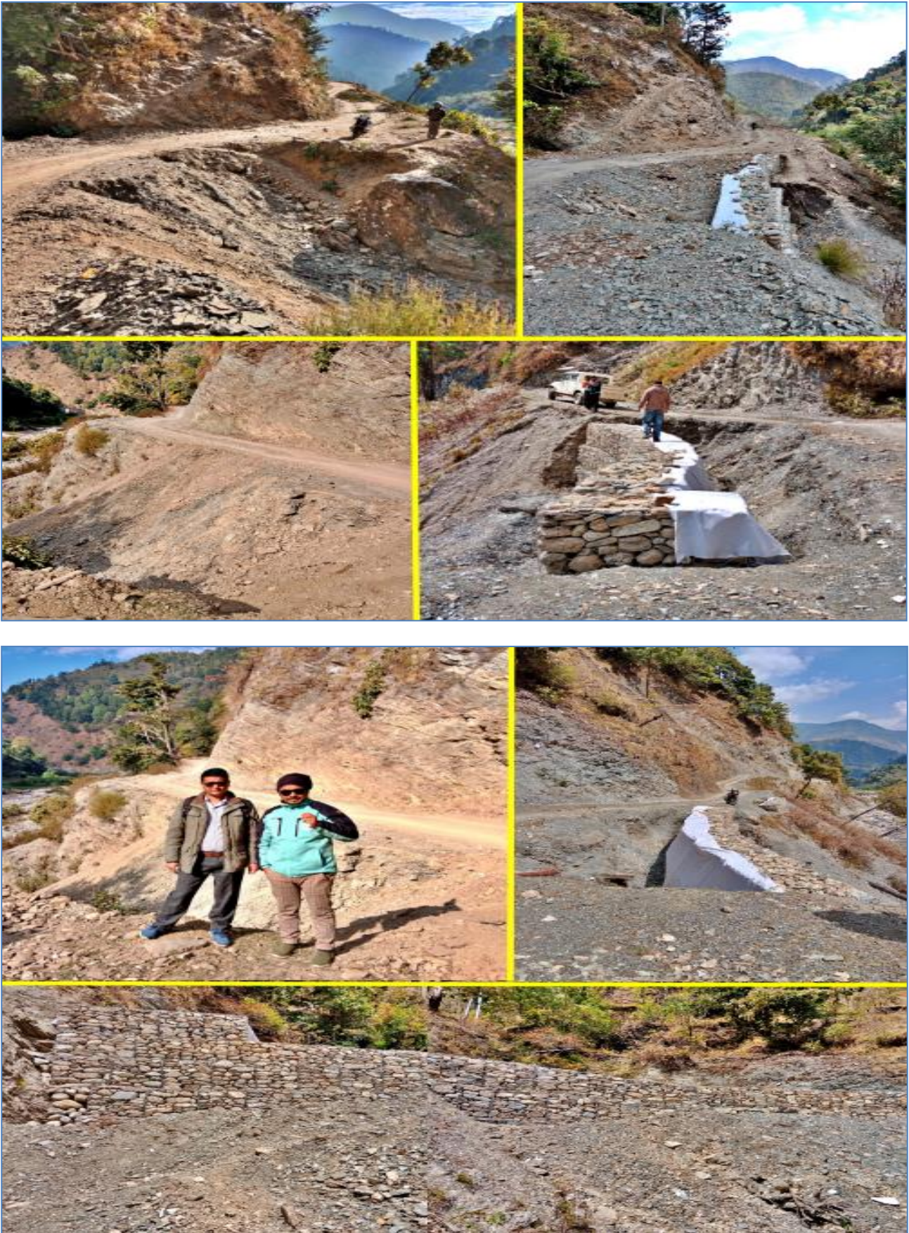
Figure 69: Balle Mairamare Rural Road Protection
