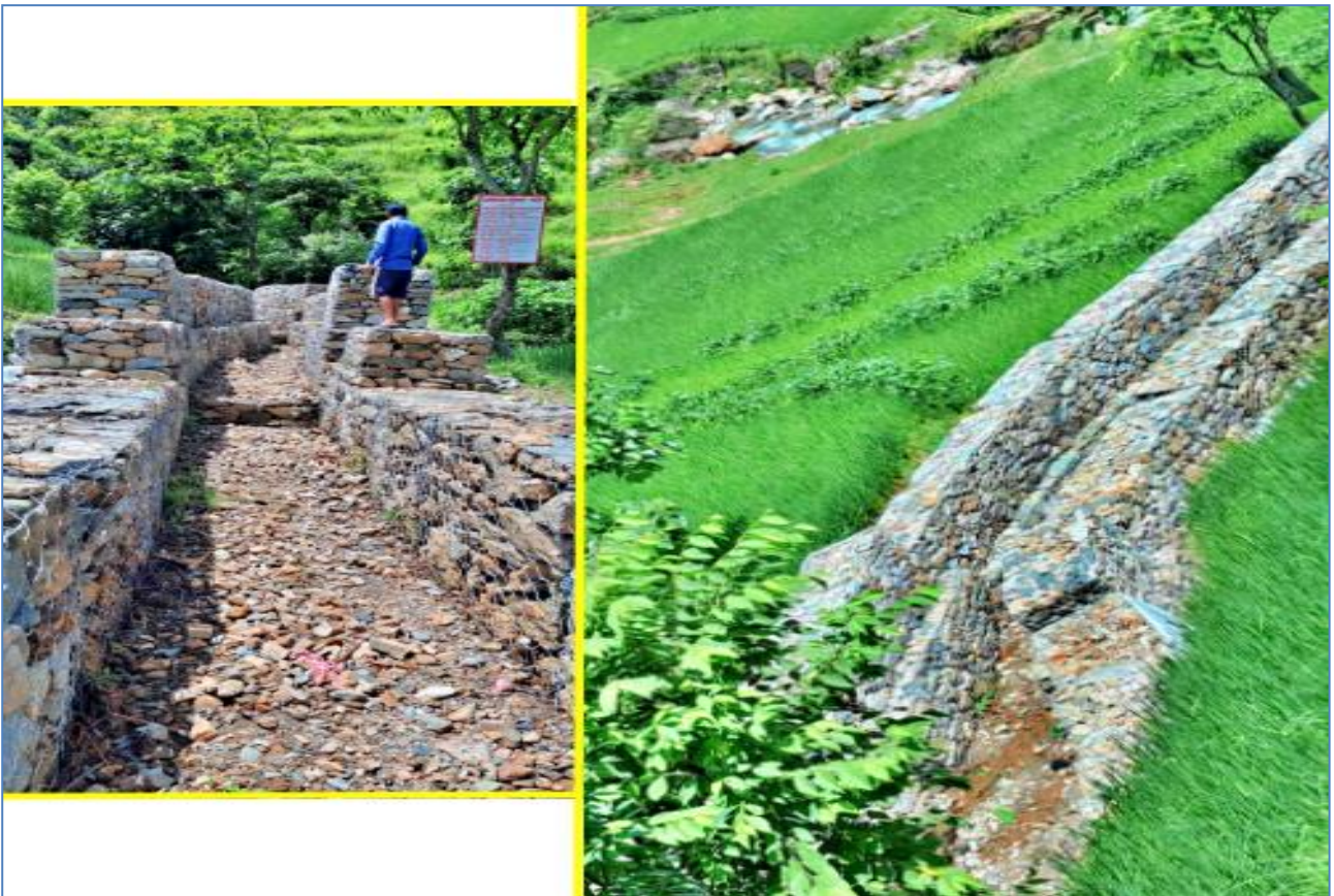
Figure 28: Jutung Khola Stream Bank Protection
