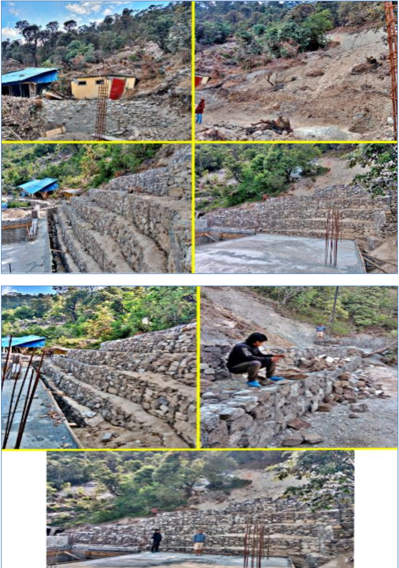
Figure 43: Kharawang Landslide Treatment
