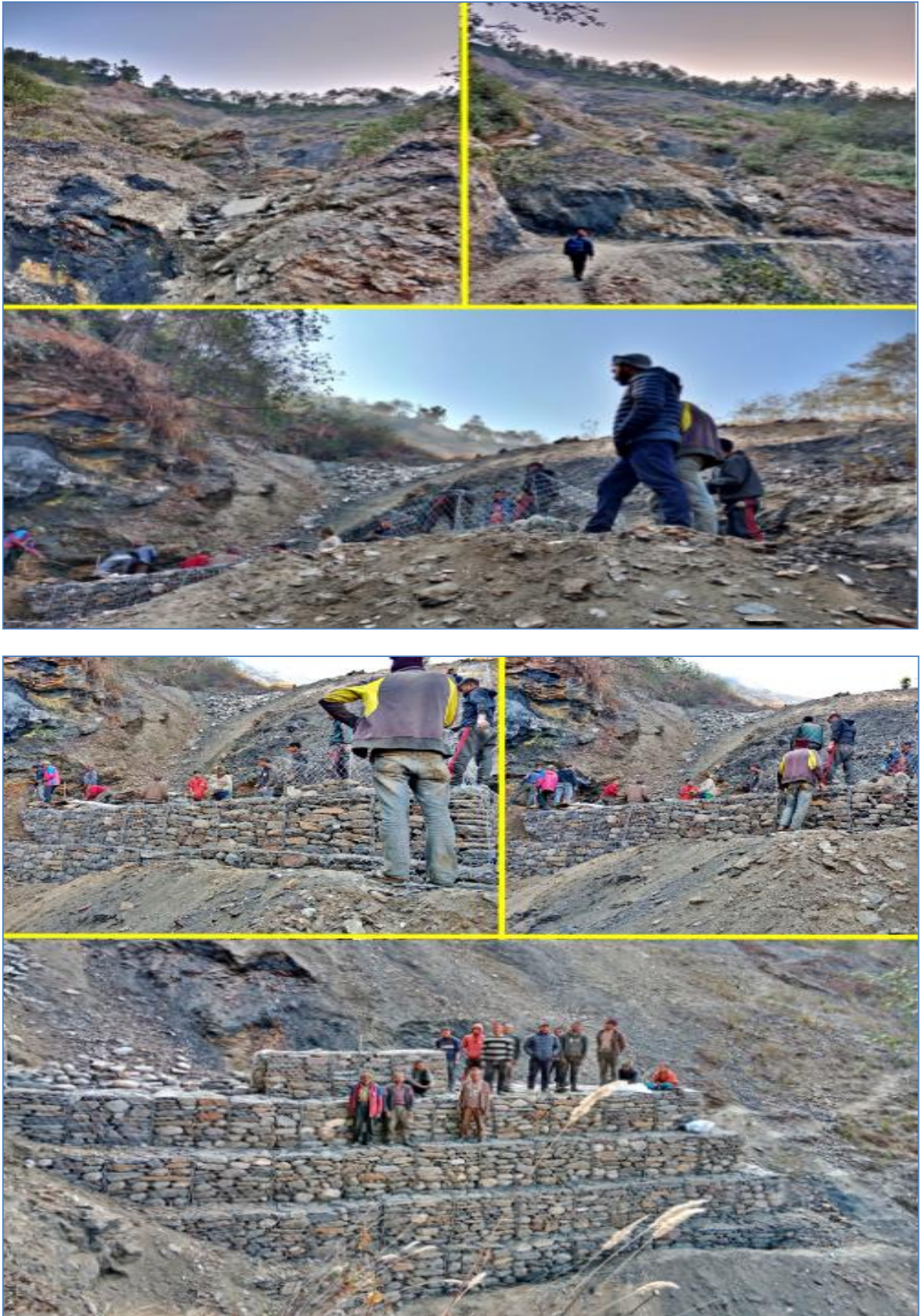
Figure 60: Dhamche Landslide Treatment
