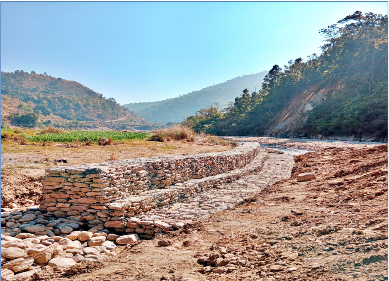
Figure 66: Todyar Arang Khola River Bank Protection
