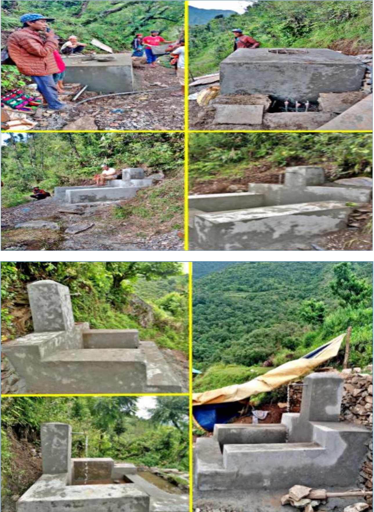
Figure 46: Daliwang Water Source Protection
