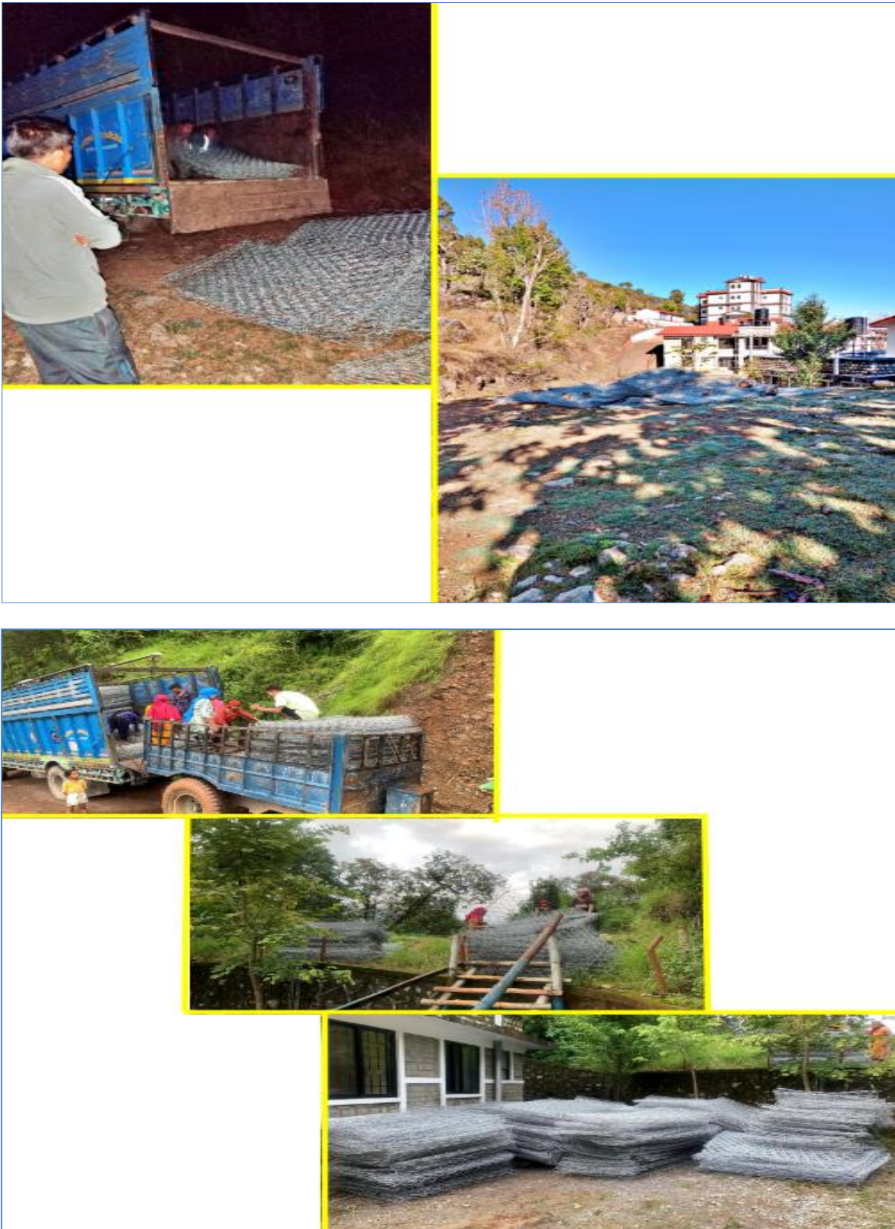
Figure 23: Gabion Boxes Procurement
