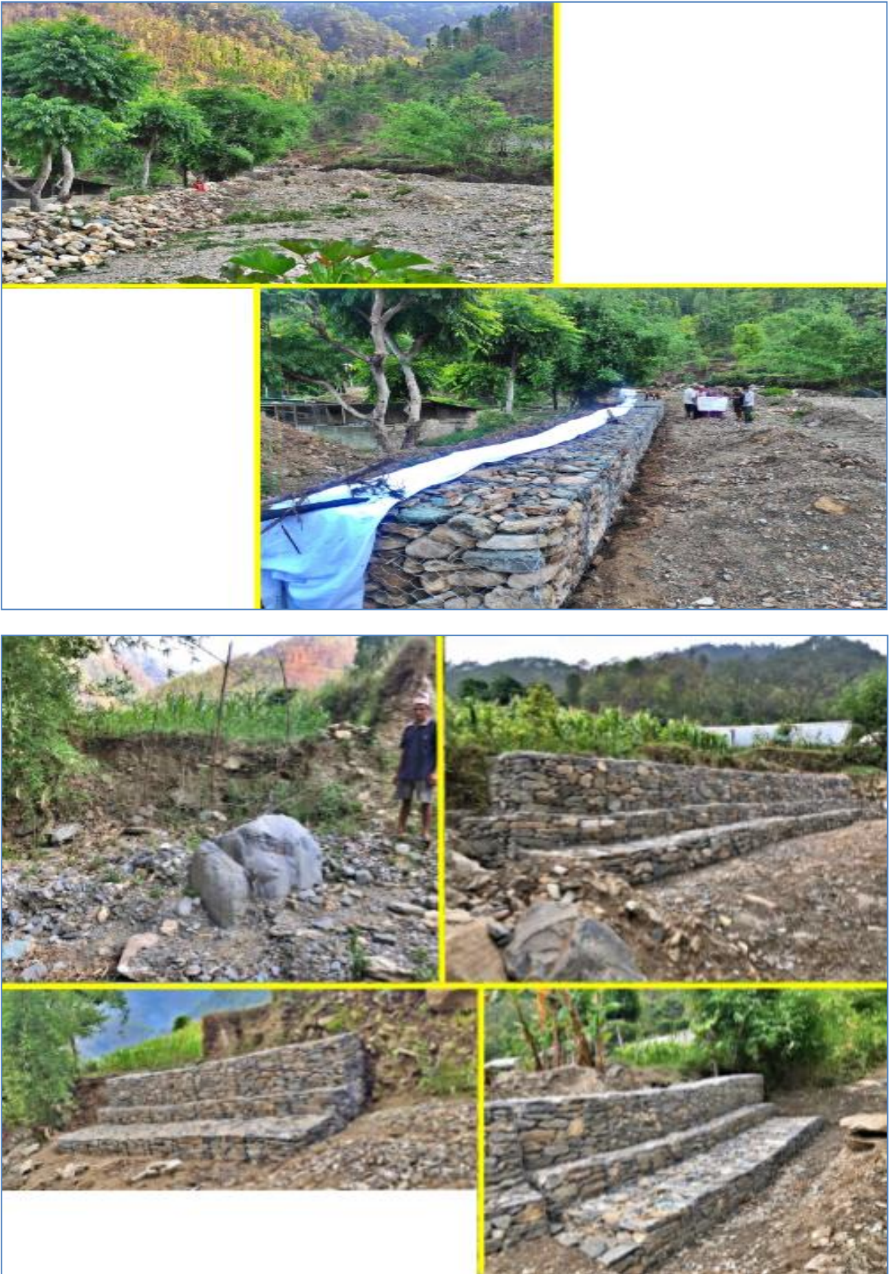
Figure 63: Chhatipata Landslide Treatment
