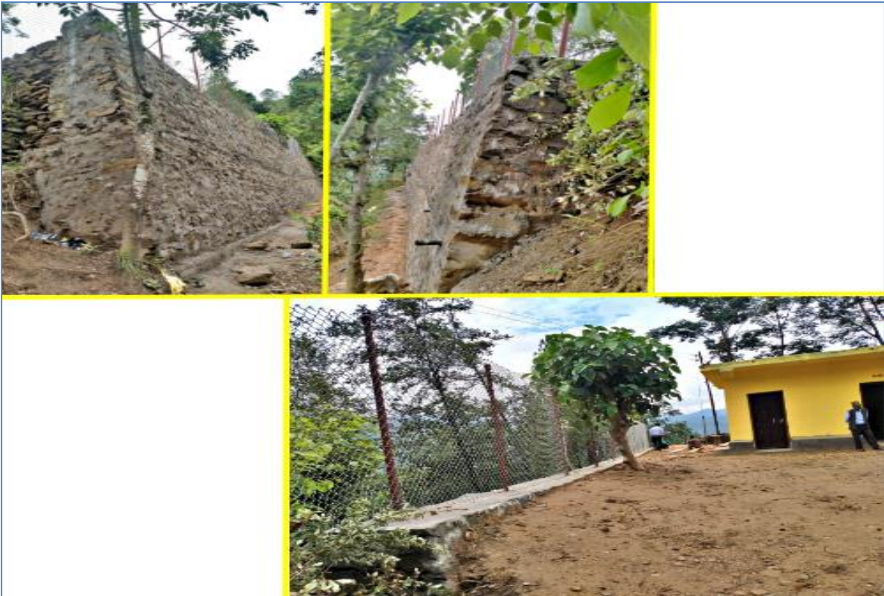
Figure 14: Simarangsi Landslide Treatment
